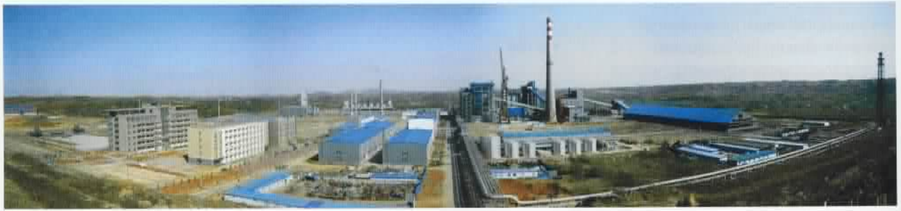
Figure 5. Yima joint venture coal-to-methanol project using SES gasification technology.
